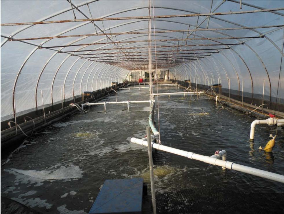
*\*A central wall divides the raceway and water is propelled around that wall by a combination of pumps and airlifts. A greenhouse structure covers the raceway to contain heat and facilitate radiant heating; this raceway is currently operated year-round.*
